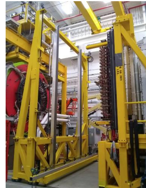
Support structure in Hall D
