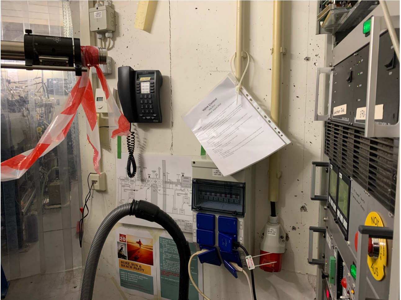
Figure 13 Telephone with number 1351, vacuum controls and sample-inlet emergency stop on right behind the beamline at the vacuum and valve control panel, close to sample inlet system. Emergency numbers 112 for ambulance or fire truck, 110 for police. The external line is connected without dialing 9! Inform the gate (3333) where the ambulance / fire truck / police are needed! You are in the Experimental hall, cave X0, EH.1.029. Send someone to green cube to guide in ambulance / fire truck.
